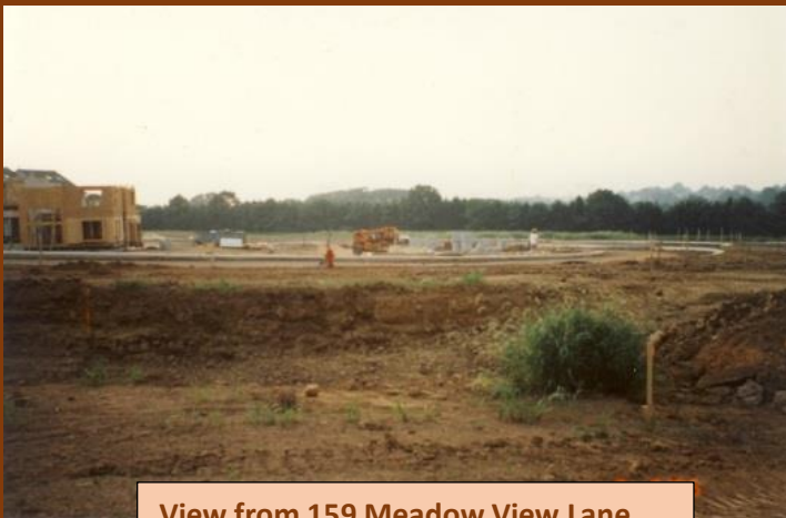
View from 159 Meadow View Lane toward 157 Center Point Lane, 8-6-96
